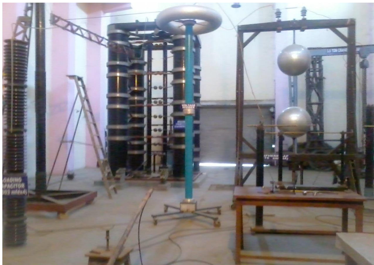
Fig.3 1.6 Million impulse voltage lab of JEC, Jabalpur where test at insulator under different level of contamination was performed
